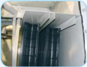
Double row high efficiency PVC drift eliminators
