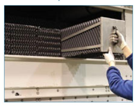
Some <u>Versapak</u> fill bundles have handles for easy removal and fill inspection! Screw-knob side access panels for fast dismantling.
